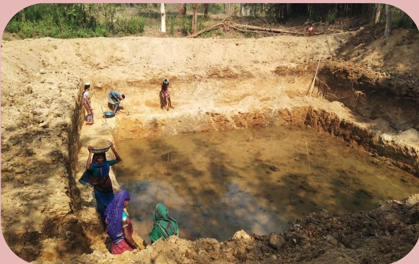
Excavation of Farm Pond at Balangir Unit
