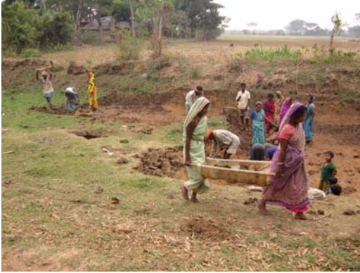
Improvised stretchers for carrying earth
