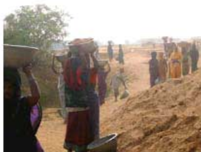
Repairing village link road through FFW scheme
