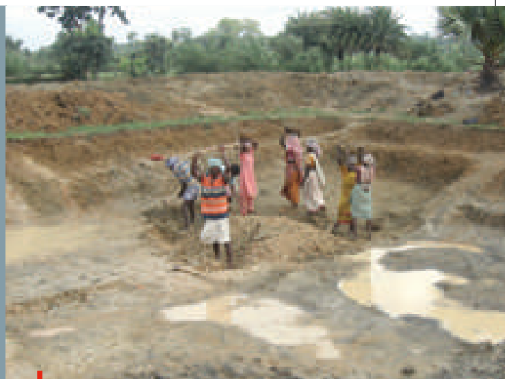
Farm pond excavation
