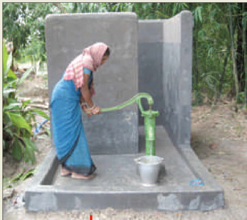
Protecting Women's Dignity Bathing Enclosure - Enables women to have adequate privacy.
