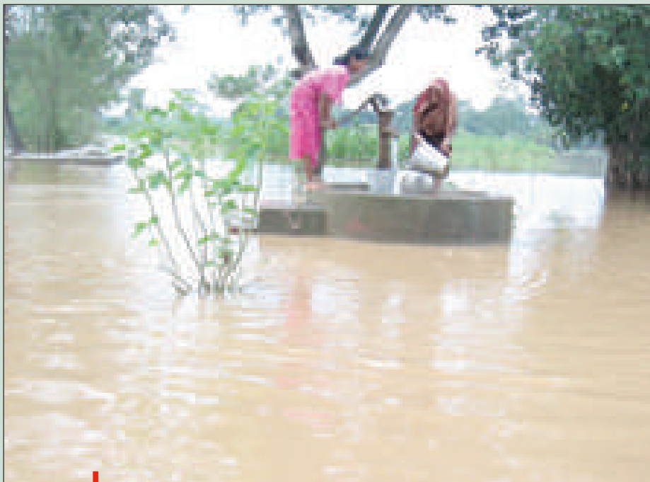
Tube well with high raised platform in a flood prone area Only source for collecting drinking water during high flood.
