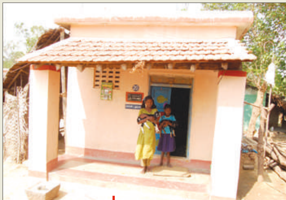
Multi hazard resistant house built in Tsunami affected areas by LWSI
