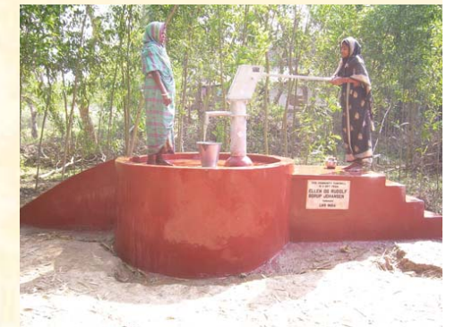
A newly installed tube well on a raised platform
