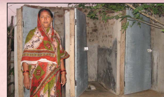
Fully constructed latrins in Krushak Bazar community promotes sanitation
