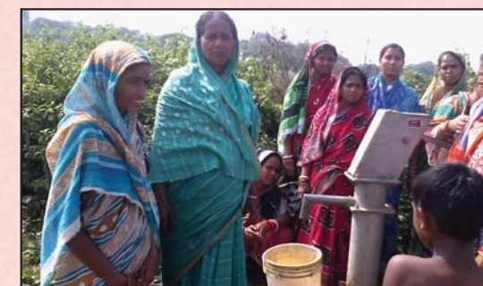
Safe drinking water source installed under the Water and Sanitation Scheme
