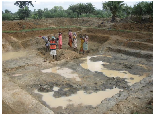
Pond Excavation for Rainwater harvesting
